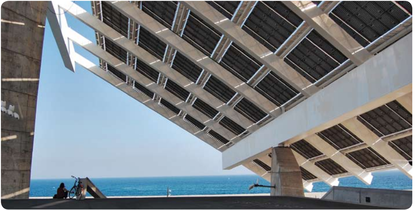
Esplanade and Photovoltaic Power Plant by racEcar_yayas/flickr.com
