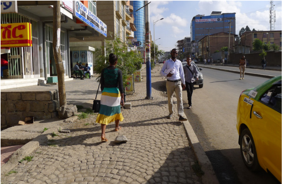
✘ The absence of a pedestrian zone forces people to walk in the carriageway. Light poles, trees, and other elements should be placed in the furniture zone.
