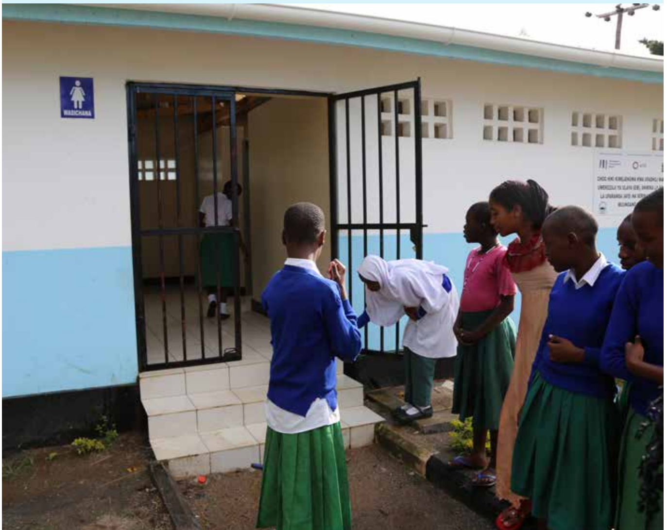
New girls toilet block. ©UN-Habitat/Julius Mwelu
