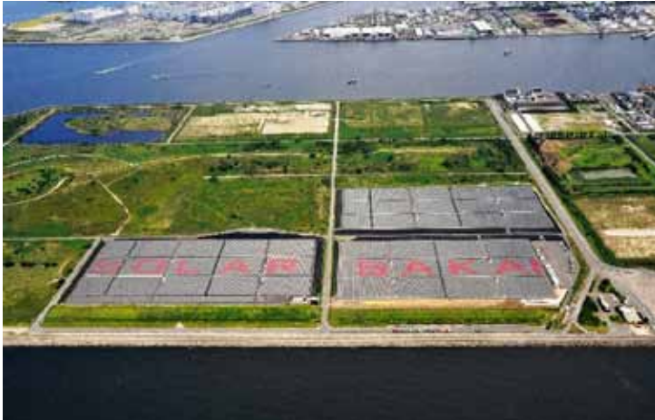
Solar power Osaka © www.osakacity.org
